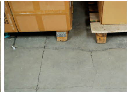
Cracked Concrete
