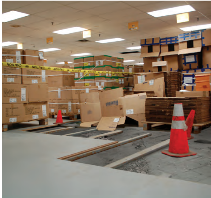
Installation of ResinDek and steel sleepers over damaged concrete.
