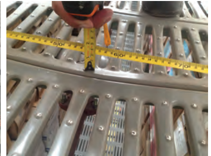
Damaged Plank Grate
