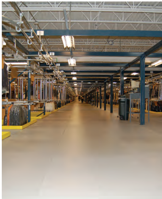
ResinDek Replaced Poly Deck at Polo Ralph Lauren
