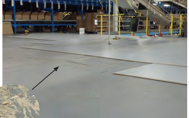
ResinDek panels over plywood is a simple affordable fix!
